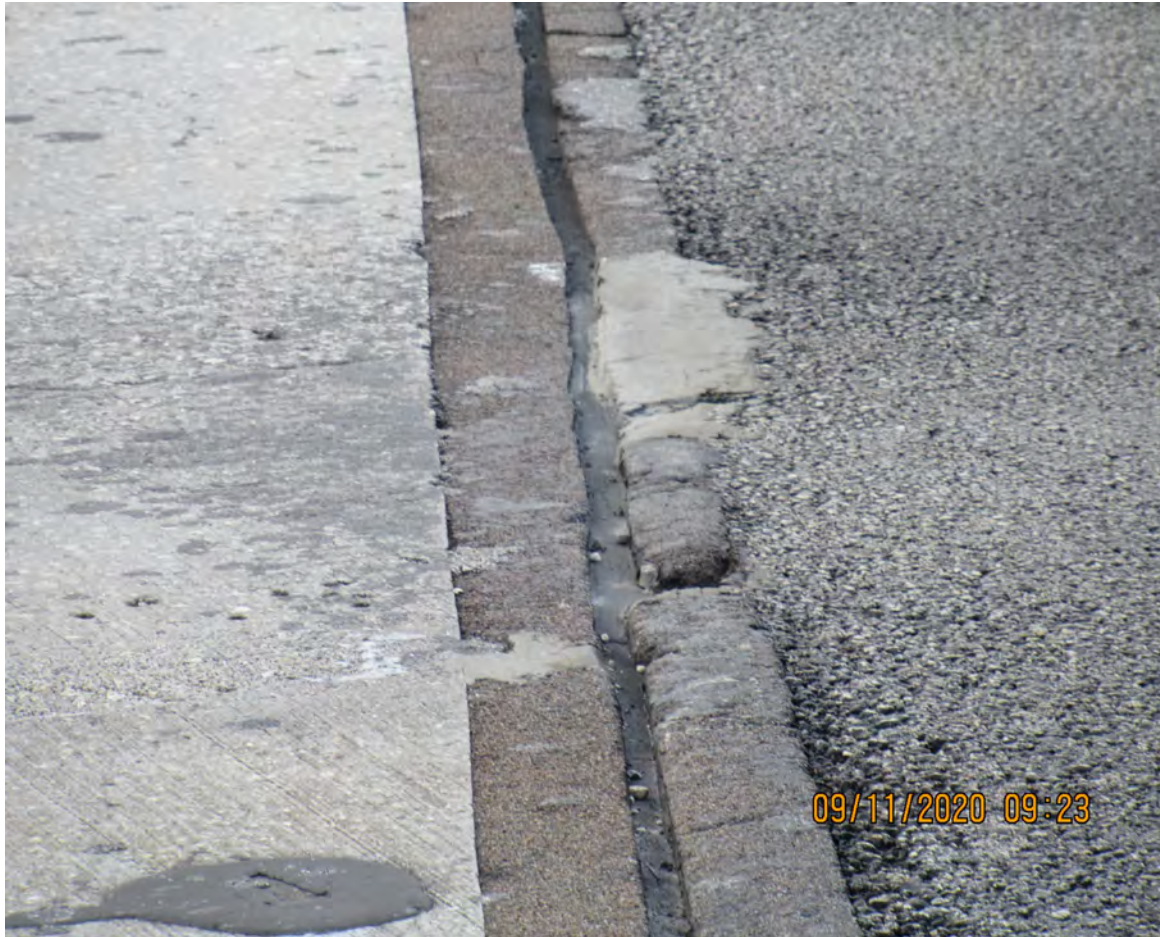
DAMAGED POLYMER NOSING JOINT HEADER (BRIDGE No. 870138)
