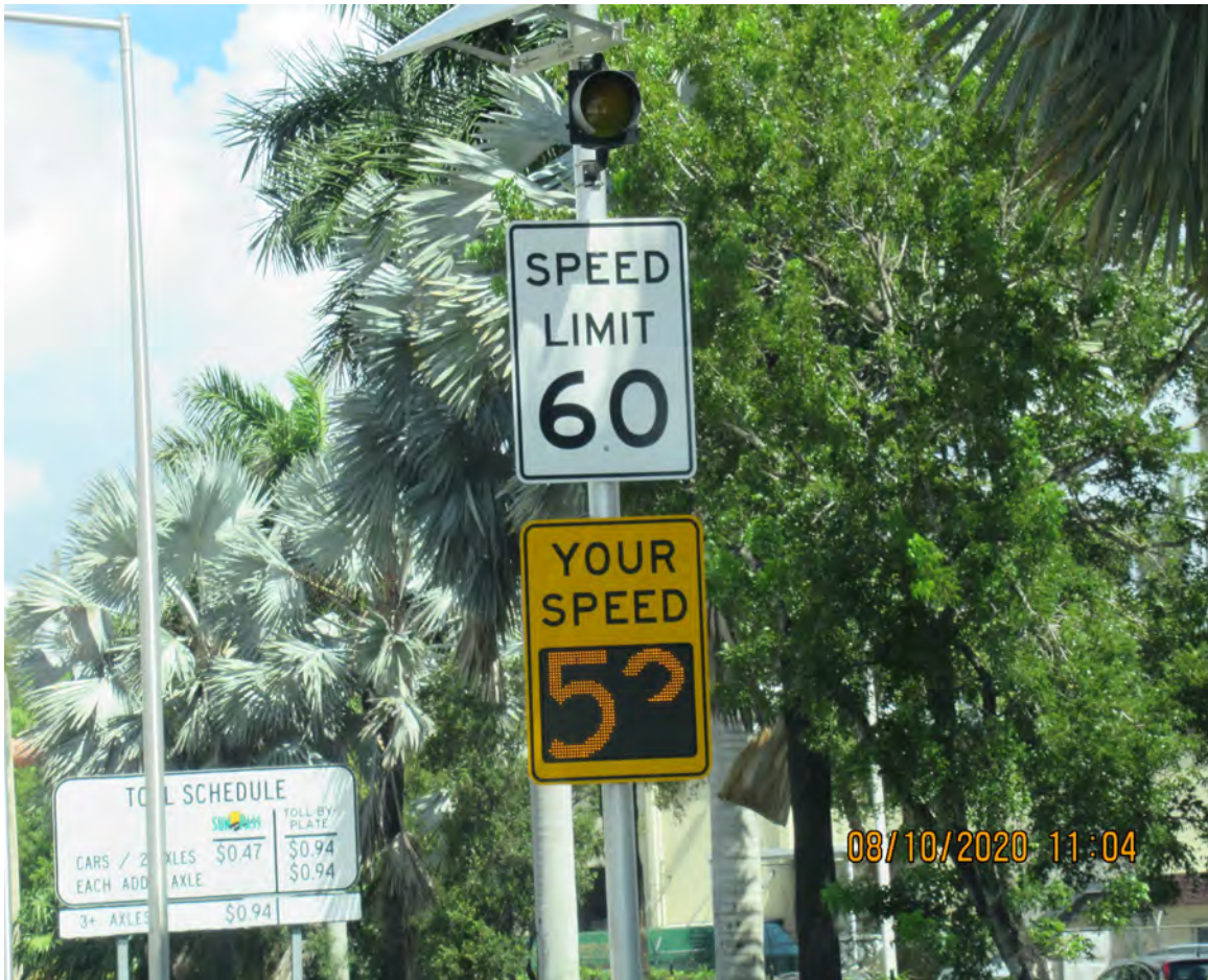
MALFUNCTIONING SPEED LIMIT SIGN
