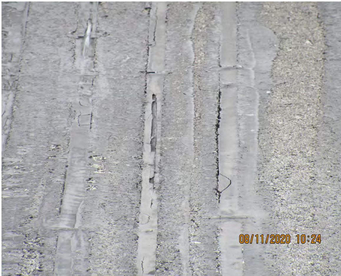
DETERIORATED TOLLS LOOP DETECTOR SEALANT
