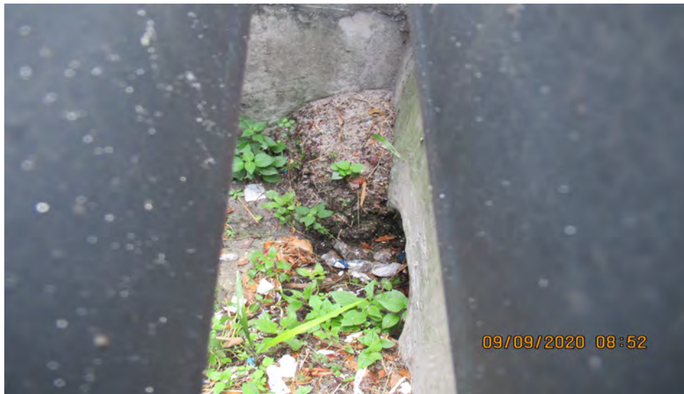
SILTED DRAINAGE INLET
