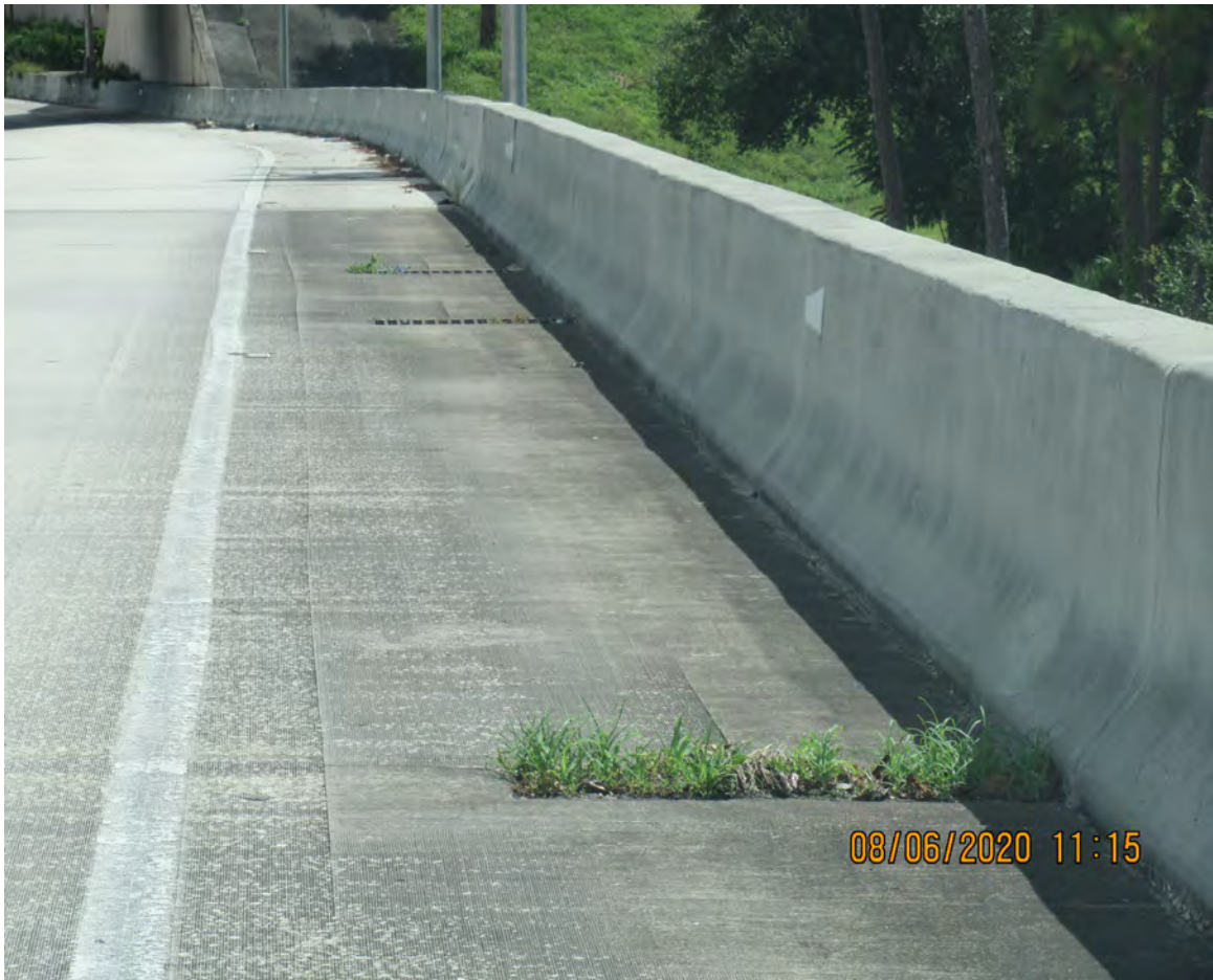
SILTED DRAINAGE INLET BRIDGE # 871024 (TYPICAL AT VARIOUS LOCATIONS)
