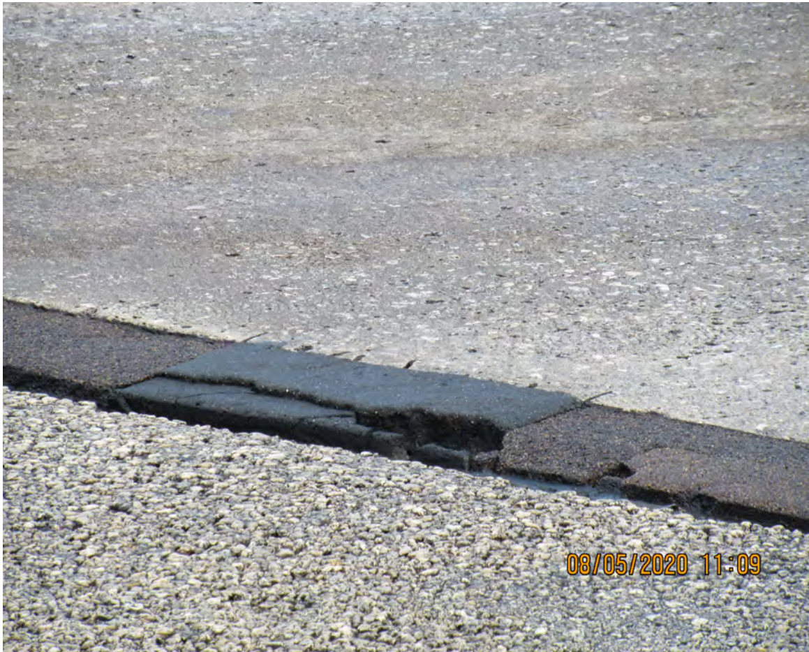
DETERIORATED POLYMER NOSING JOINT HEADER (BRIDGE # 870462)
