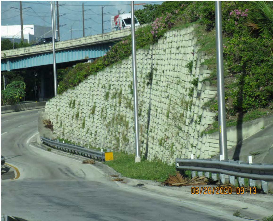
VEGETATION ON RETAINING WALL
