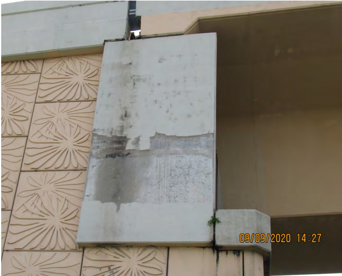
DETERIORATED CLASS V COATING ON WING WALL AT BENT 12 (BRIDGE # 871050)
