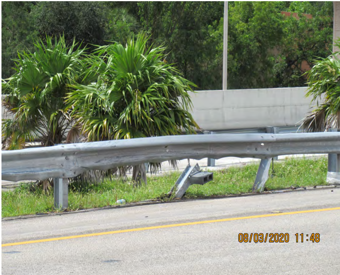
DAMAGED GUARDRAIL & GUARDRAIL POST
