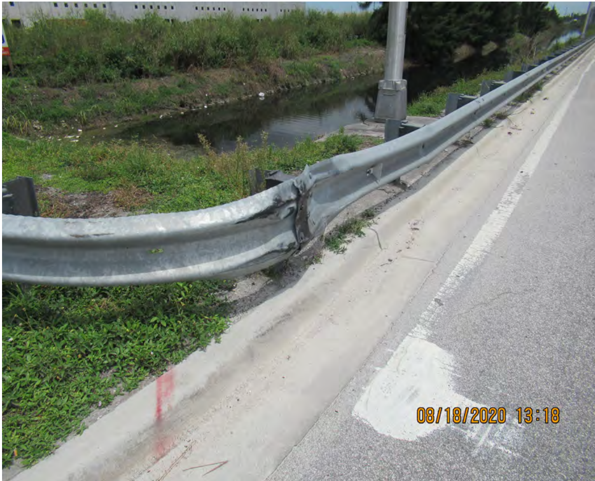
DAMAGED GUARDRAIL PANELS
