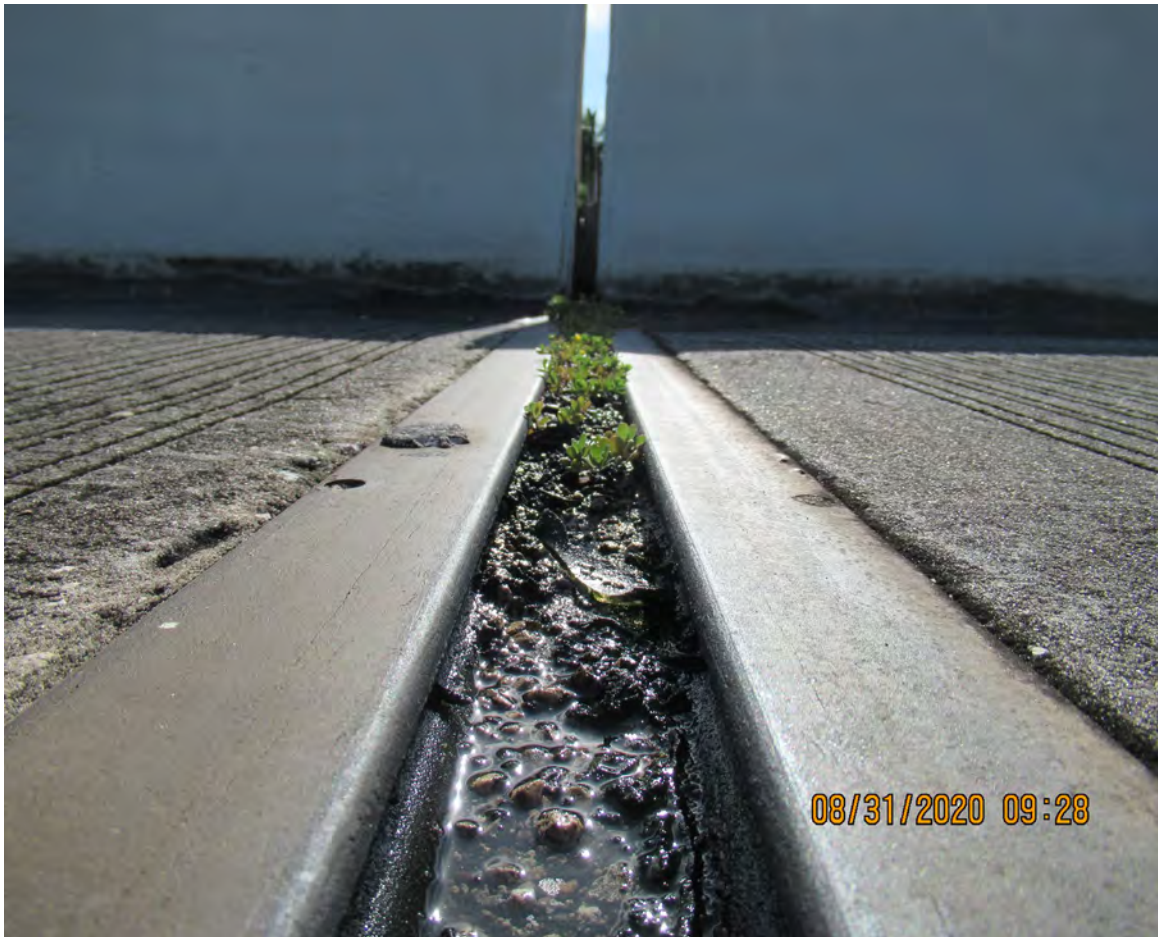
SILT AND DEBRIS ON BRIDGE JOINTS (BRIDGE No. 870725)
