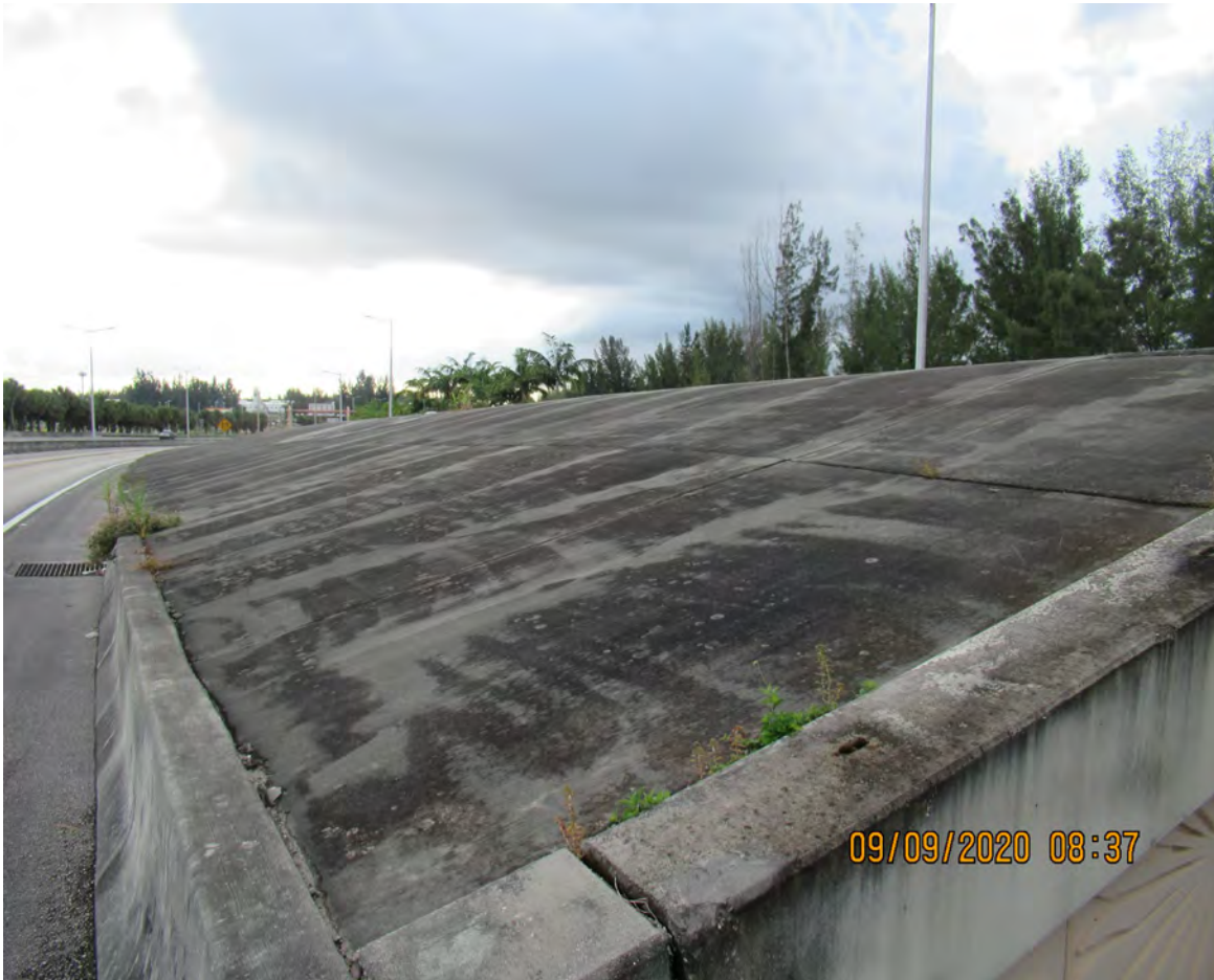
DETERIORATED CLASS V COATING ON CONCRETE MEDIAN
