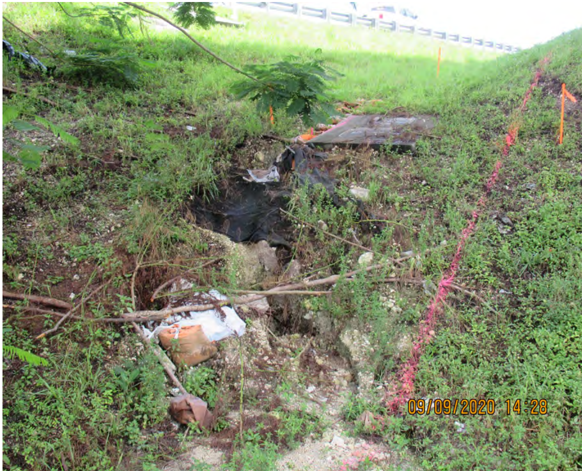
EROSION ON SLOPE (BRIDGE 871050 Span 11)
