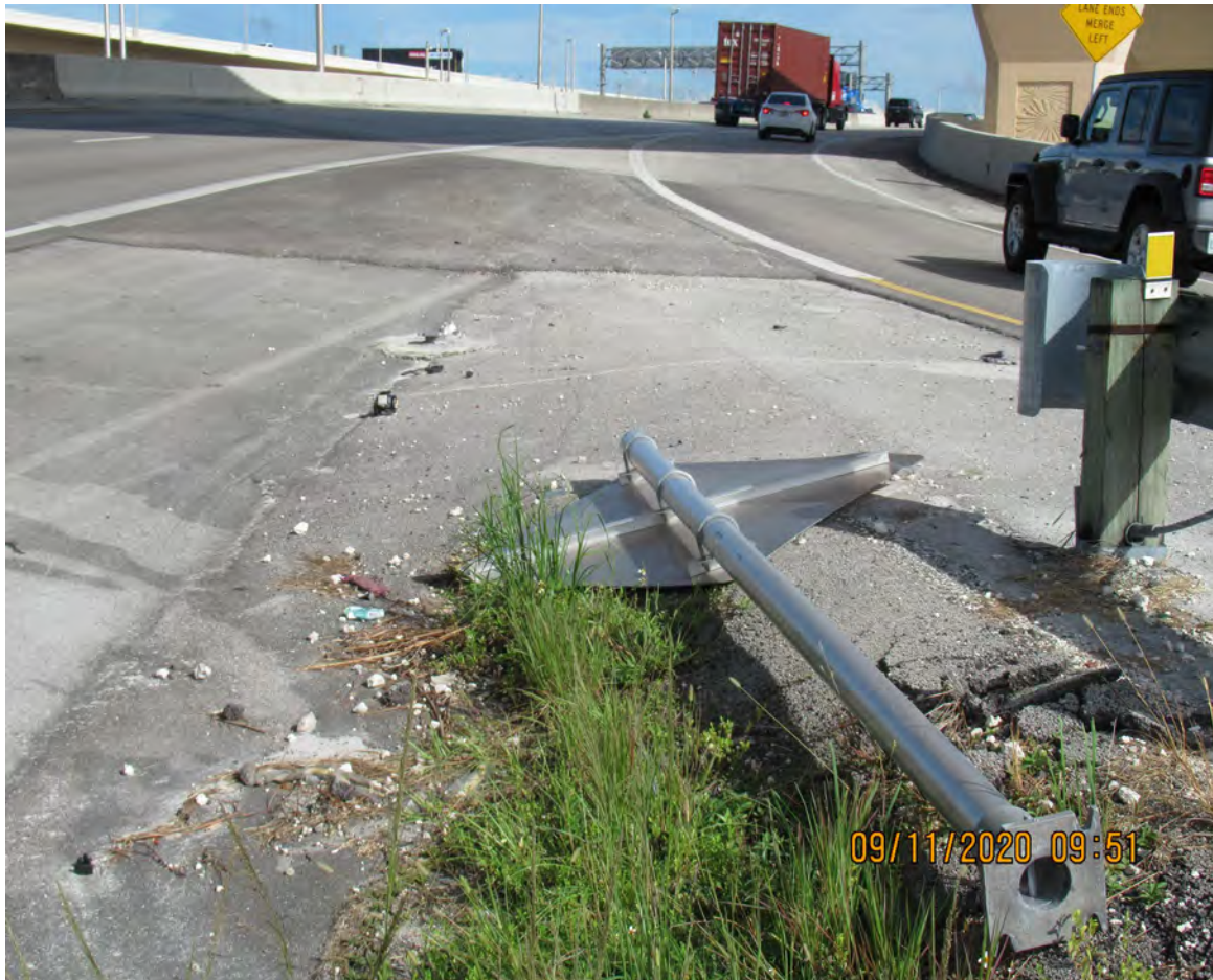
DOWN MERGE SIGN DUE TO VEHICULAR ACCIDENT
