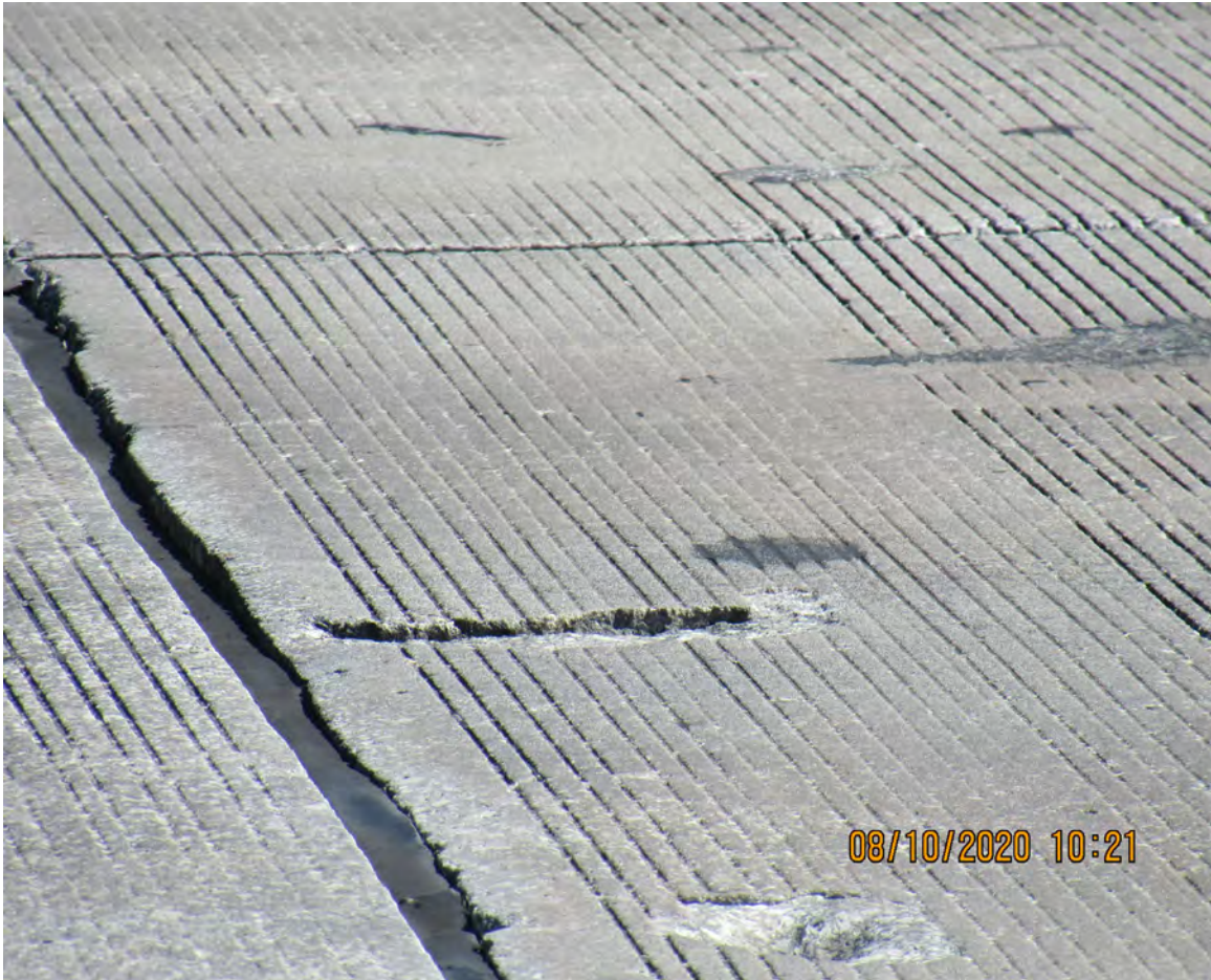
SPALLS ON APPROACH SLAB (BRIDGE # 870721)
