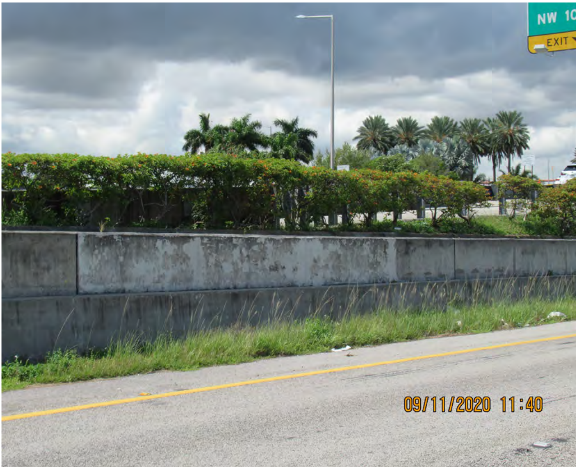
DETERIORATED CLASS V COATING ON RETAINING WALL
