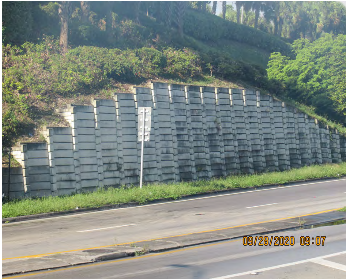
DETERIORATED CLASS V COATING ON RETAINING WALL
