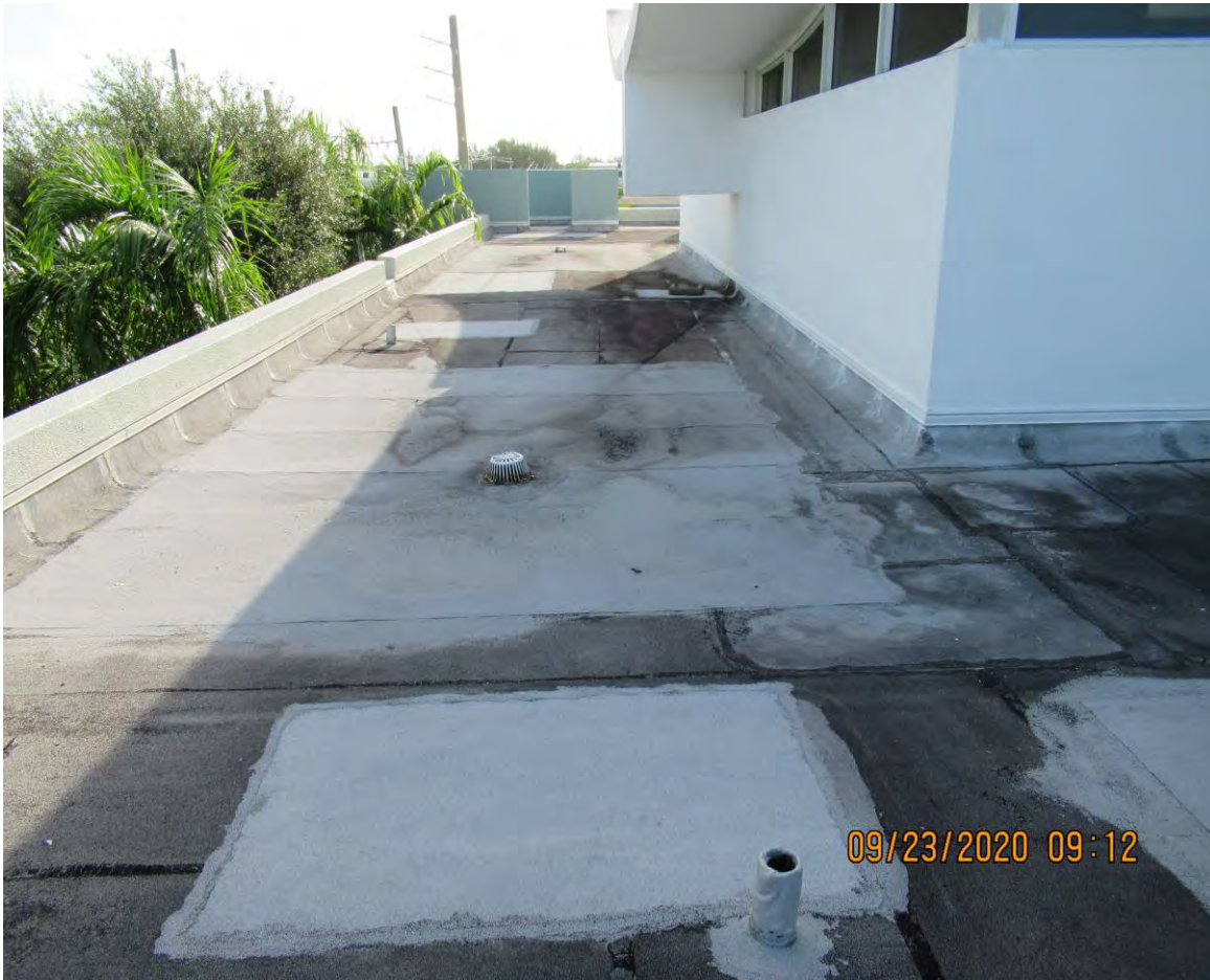
ISOLATED REPAIRS ON ROOF MEMBRANE
