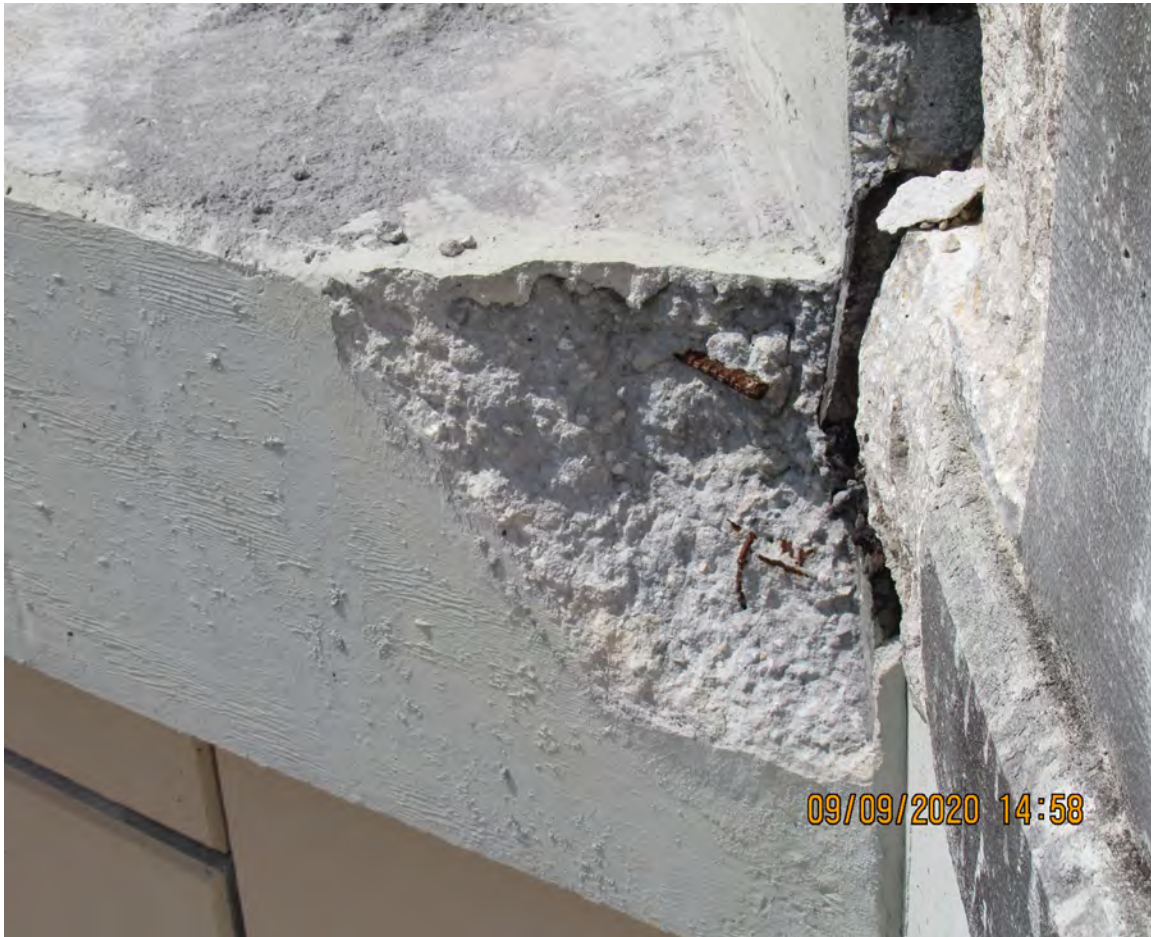
SPALL ON ABUTMENT 1 (BRIDGE # 870966)
