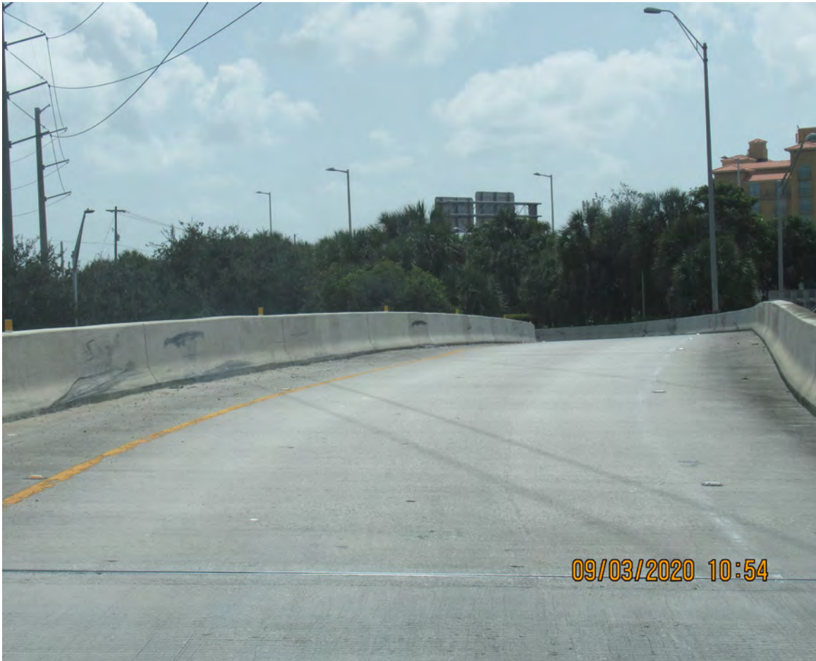
DETERIORATED STRIPING ON BRIDGE No. 870962
