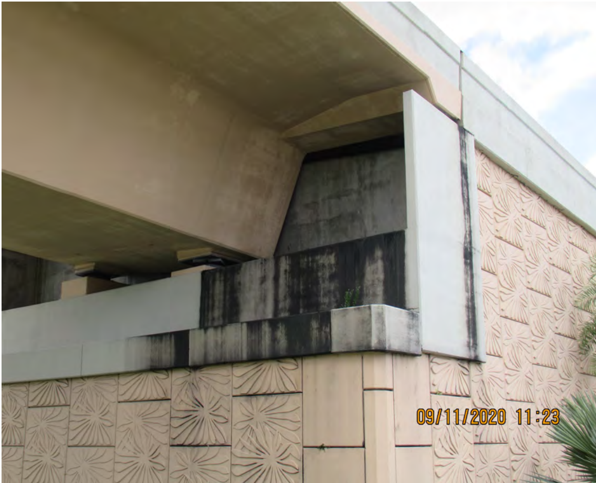
WATER STAINS FROM CLOGGED BRIDGE DRAINAGE (BRIDGE # 871046)
