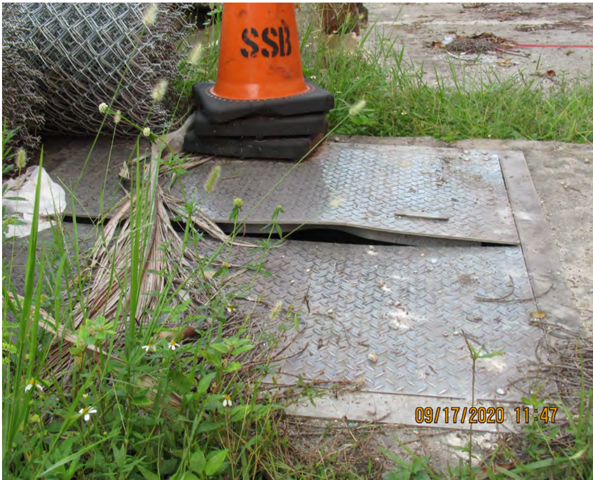
DAMAGED SPLICE VAULT ACCESS PLATE
