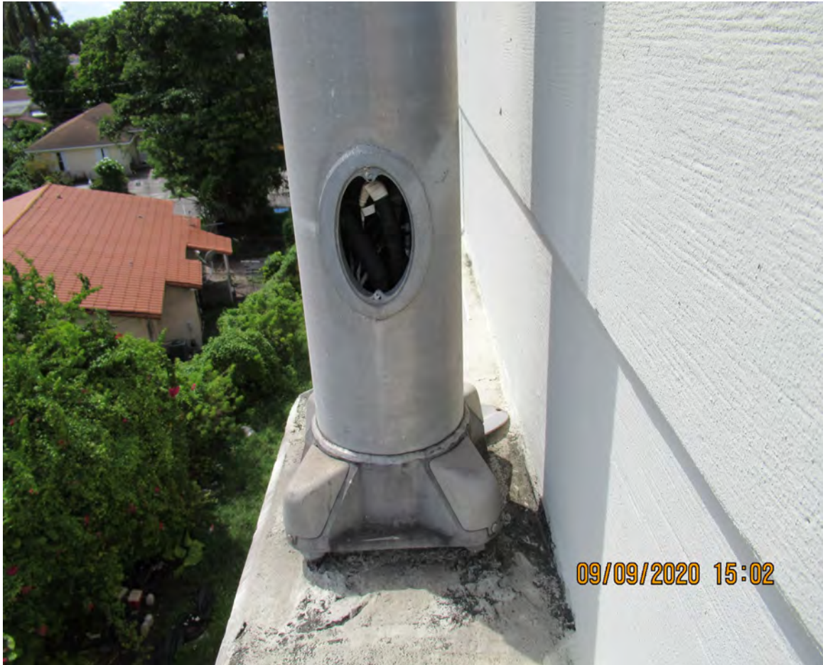
MISSING HANDHOLE COVER (POLE ID # 11-9A-1-2)
