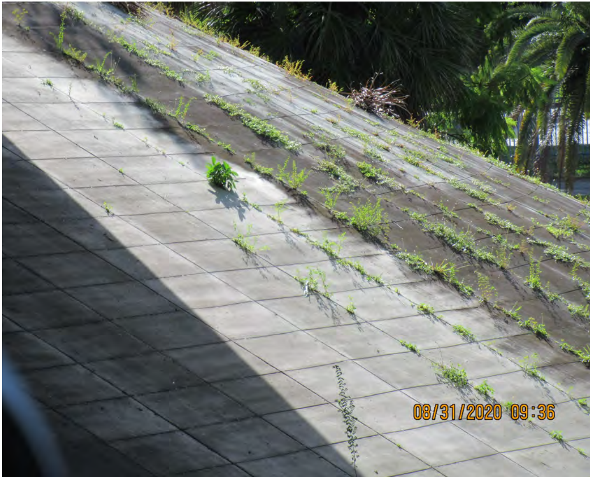
OVERGROWN VEGETATION ON BRIDGE SLOPE (BRIDGE # 870024)
