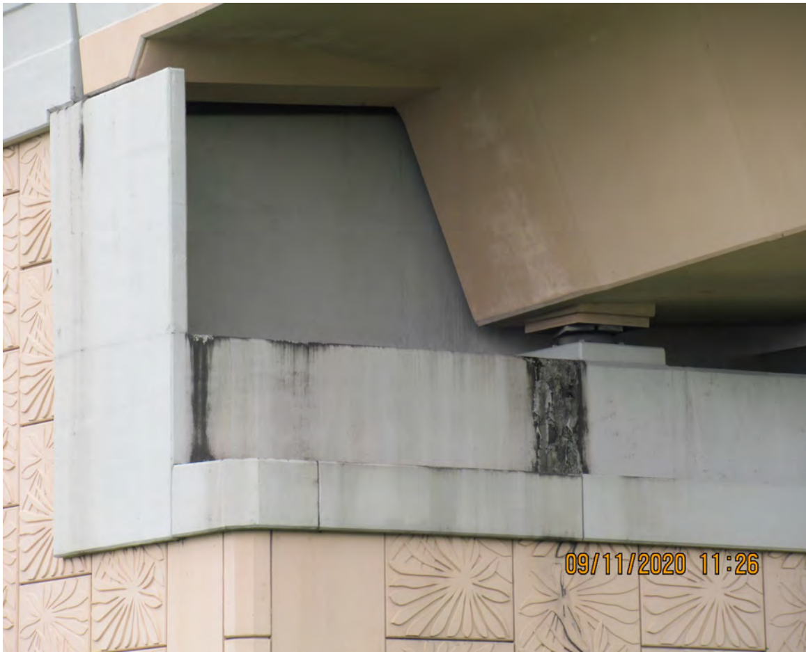
WATER STAINS FROM CLOGGED BRIDGE DRAINAGE (BRIDGE # 870078)
