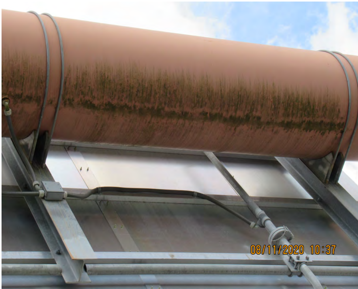
DETERIORATED PAINT ON SIGN STRUCTURE MONOTUBE (STRUCTURE # 87A053)
