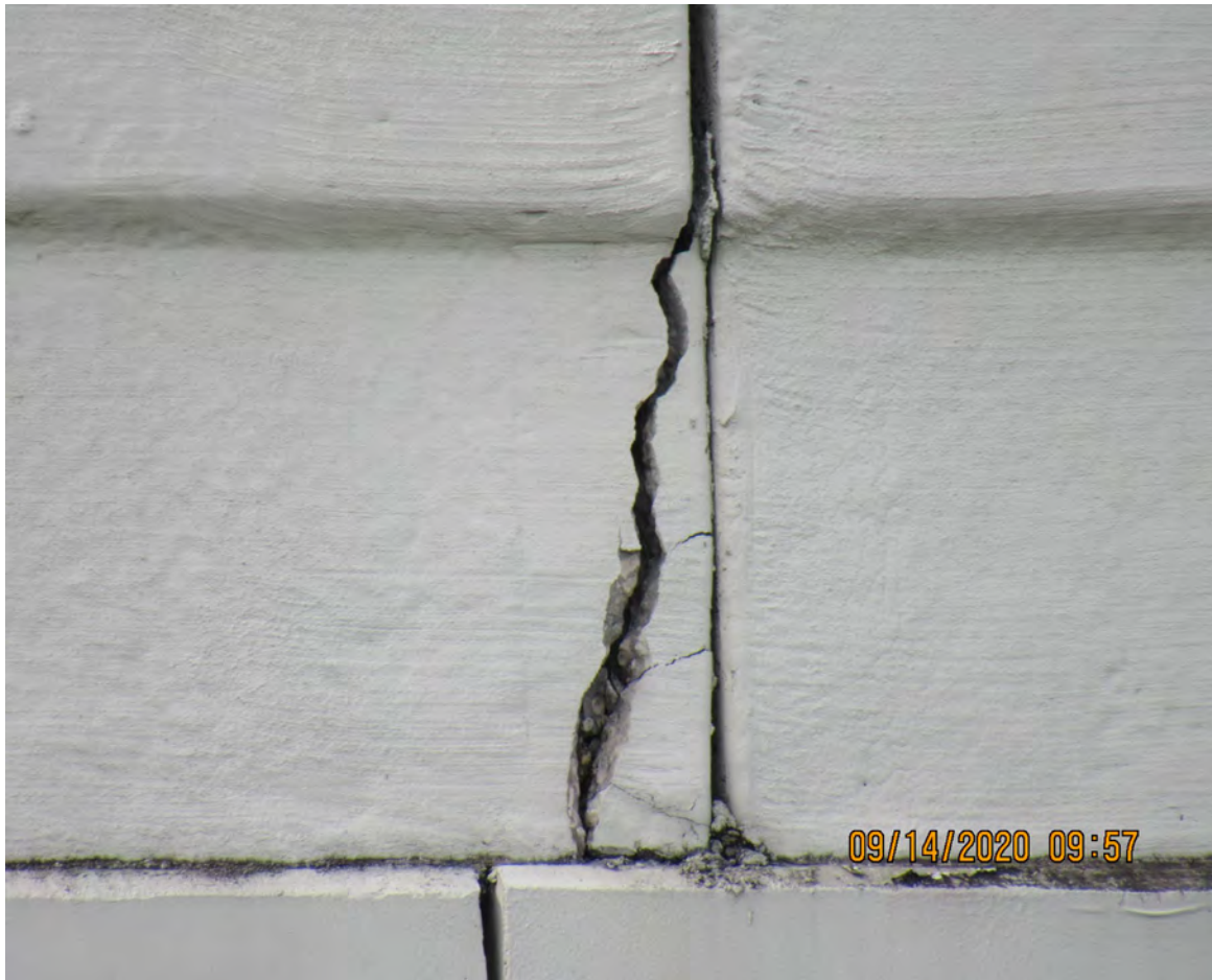
CRACKED BARRIER WALL
