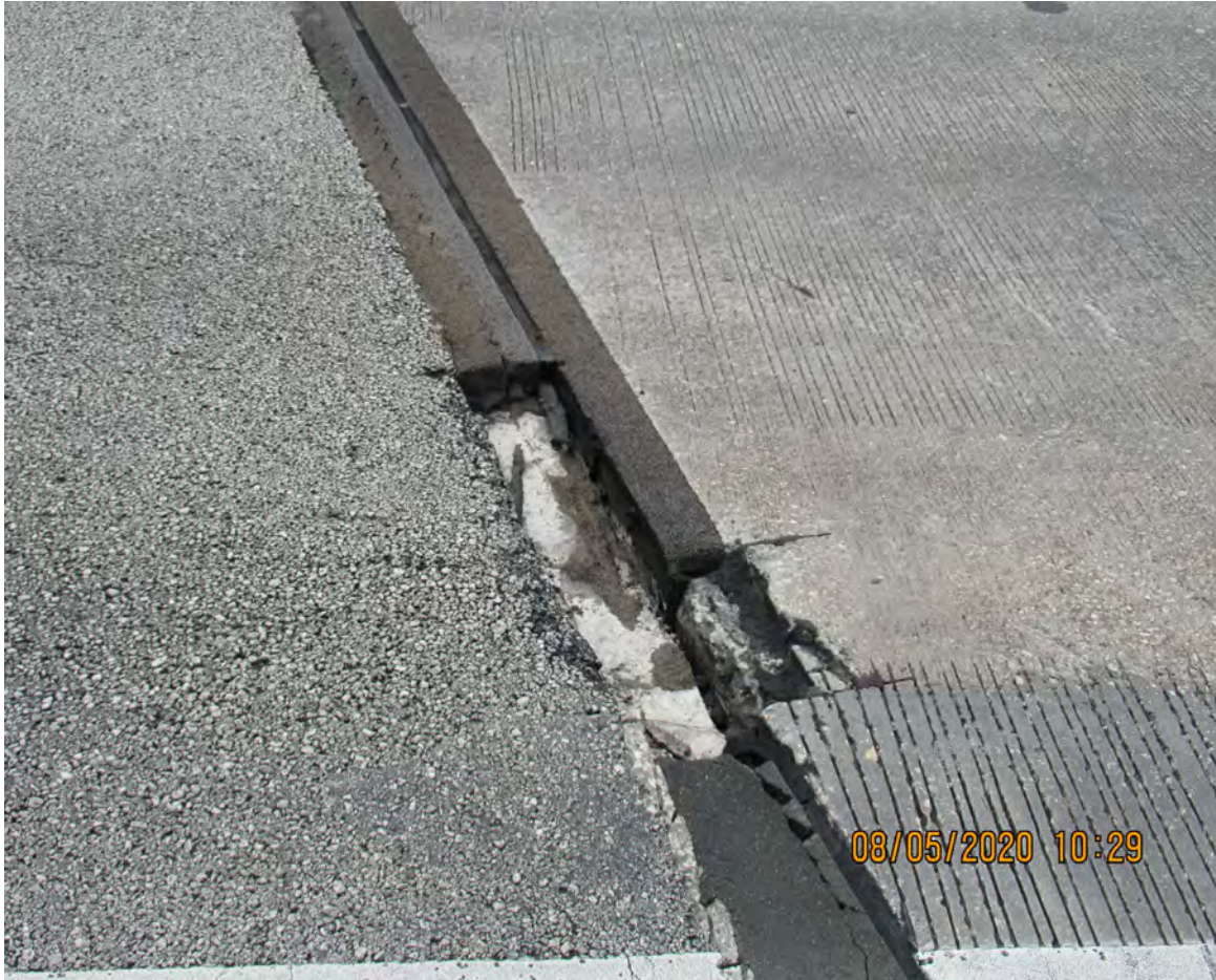
DAMAGED POLYMER NOSING JOINT HEADER (BRIDGE # 870495)
