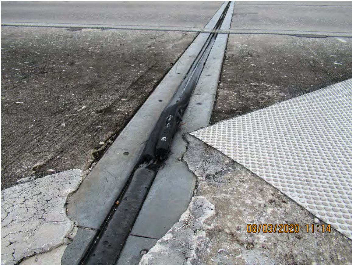
DETERIORATED EXPANSION JOINTS (BRIDGE #870557) TYPICAL THROUGHOUT THE CORRIDOR
