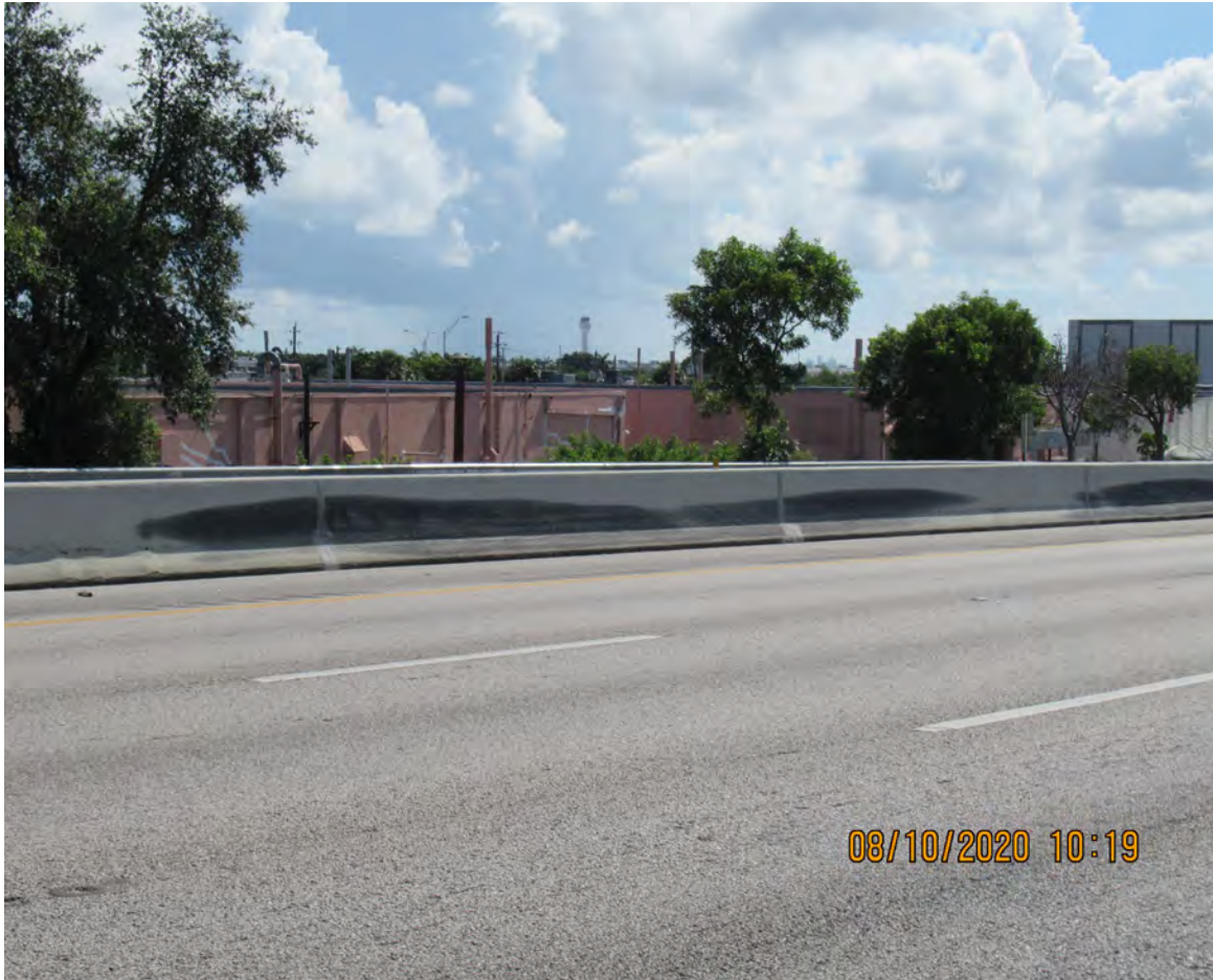
SCUFF MARKS ON MEDIAN BARRIER WALL (TYPICAL THROUGHOUT THE CORRIDOR)
