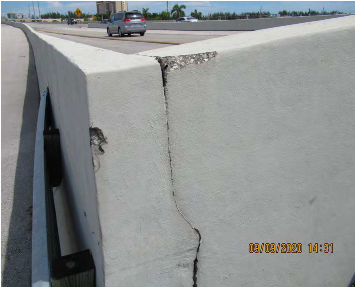
SPALLS ON BARRIER WALL
