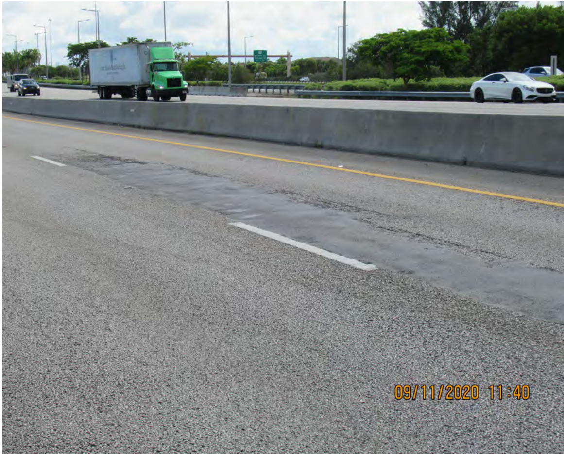
DETERIORATED ASPHALT REPAIR
