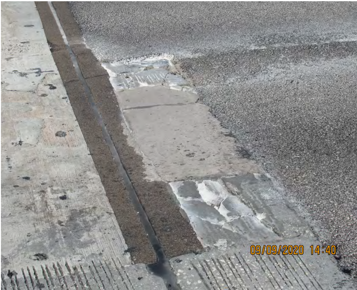
DETERIORATED APPROACH SLAB REPAIR
