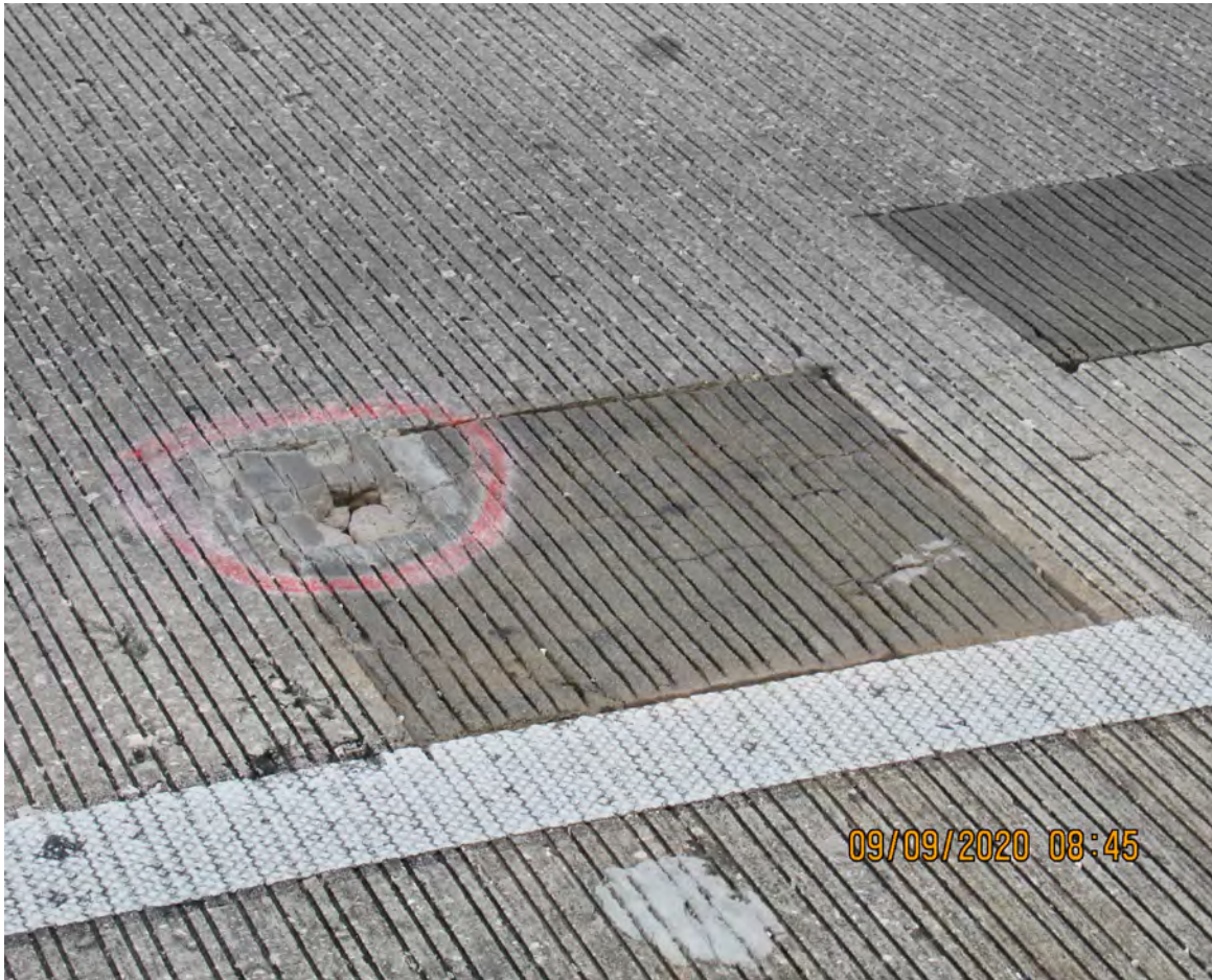
SPALL ON BRIDGE DECK (BRIDGE No. 871002)
