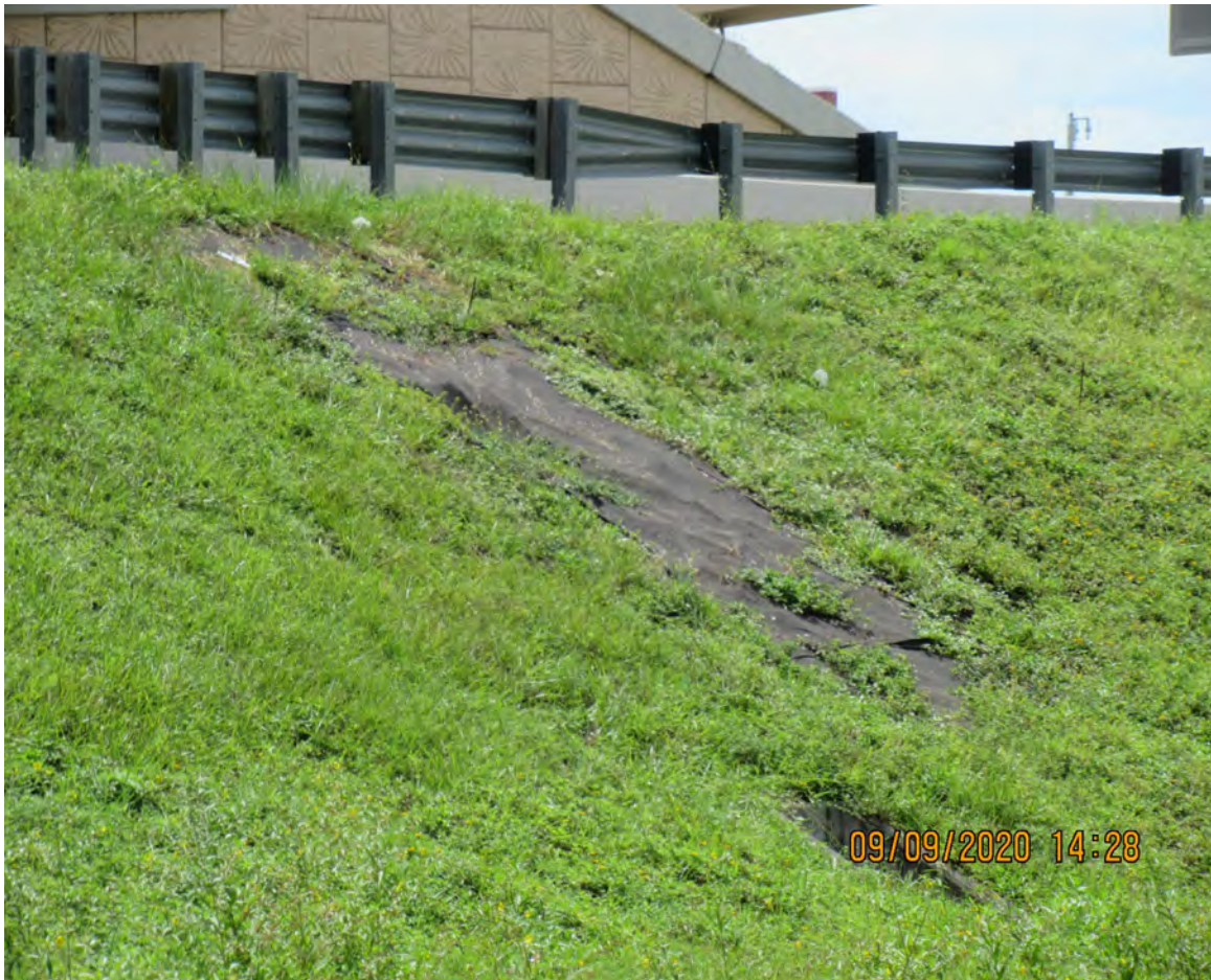
EROSION ON SLOPE (UNDERNEATH BRIDGE No. 871050 SPAN 11)
