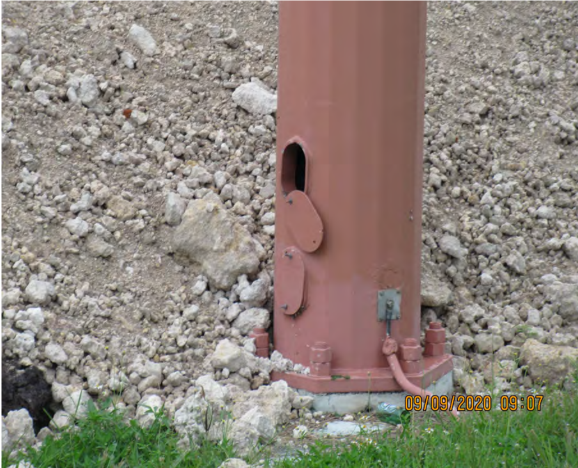
OPEN HANDHOLE ON HIGH-MAST POLE
