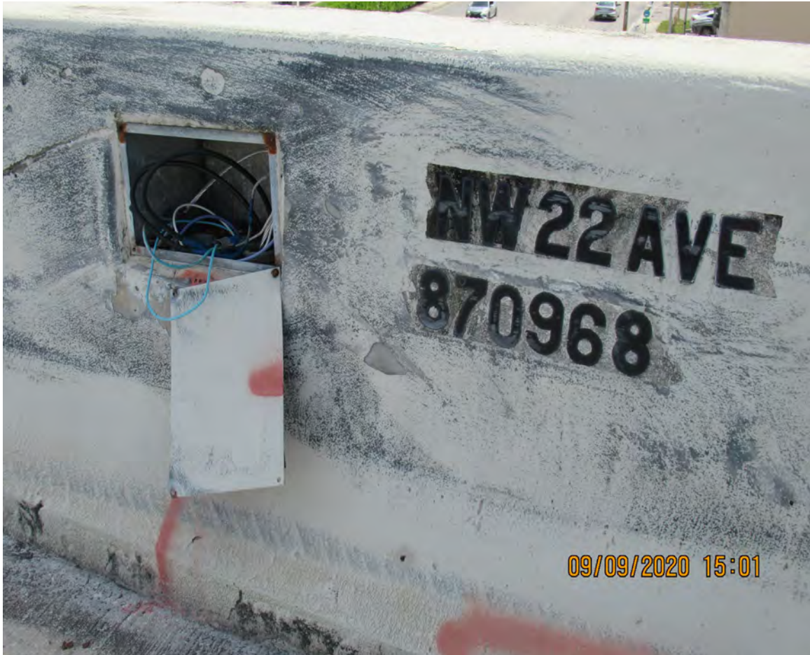
DETACHED PULL BOX COVER (BRIDGE # 870968)
