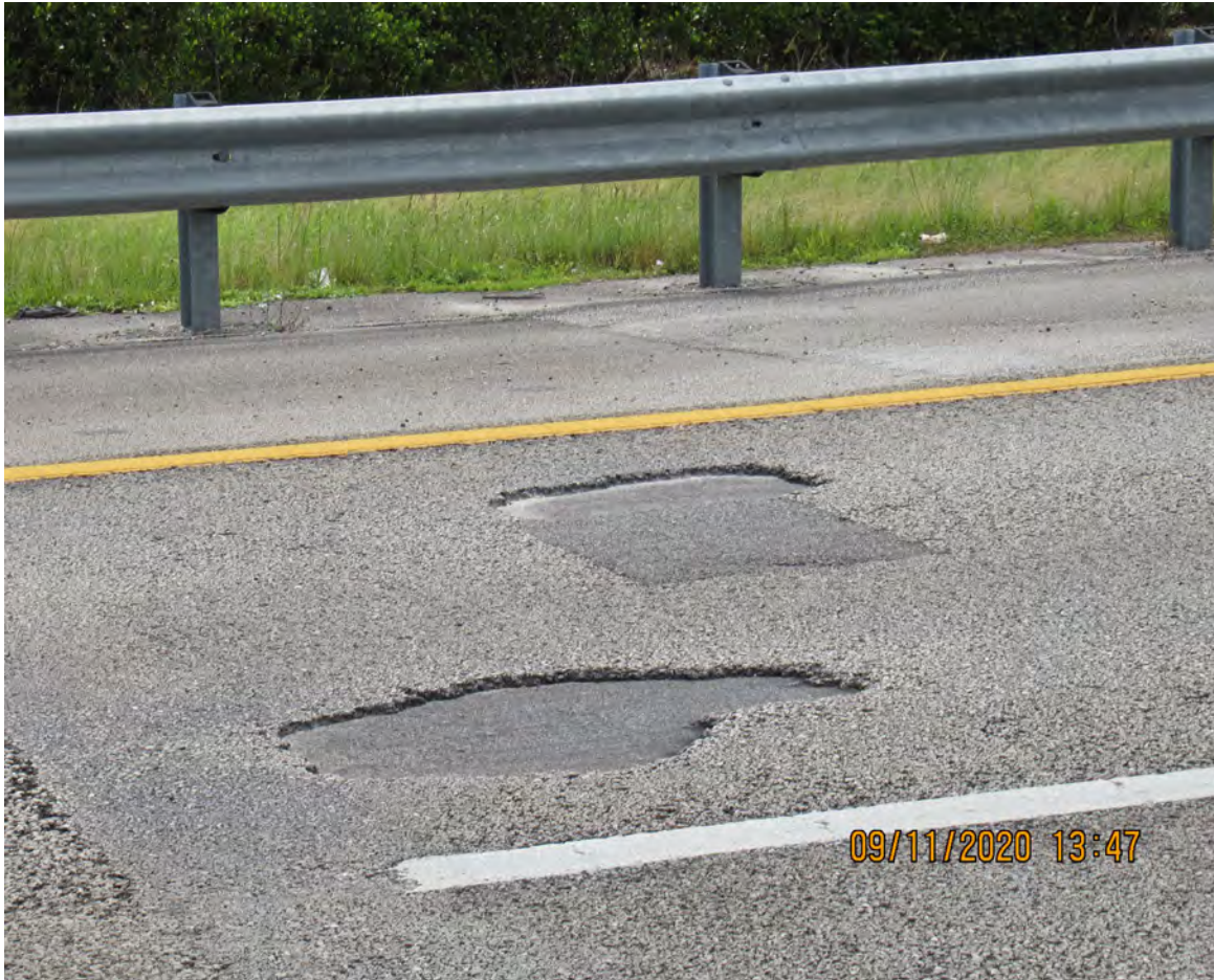
DAMAGED ASPHALT PAVEMENT FRICTION COURSE
