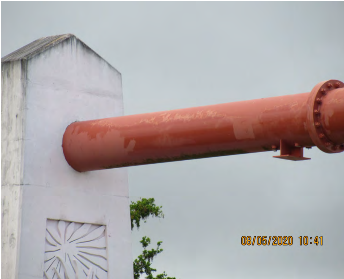
DETERIORATED PAINT ON ORT GANTRY MONOTUBE STRUCTURE
