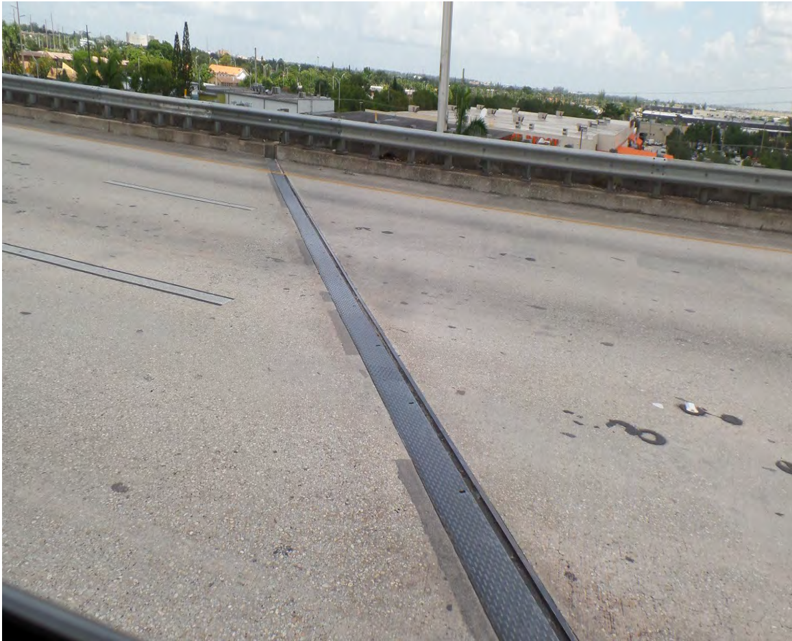
SLIDING PLATE EXPANSION JOINT BRIDGE # 870238 (TYPICAL AT VARIOUS LOCATIONS)
