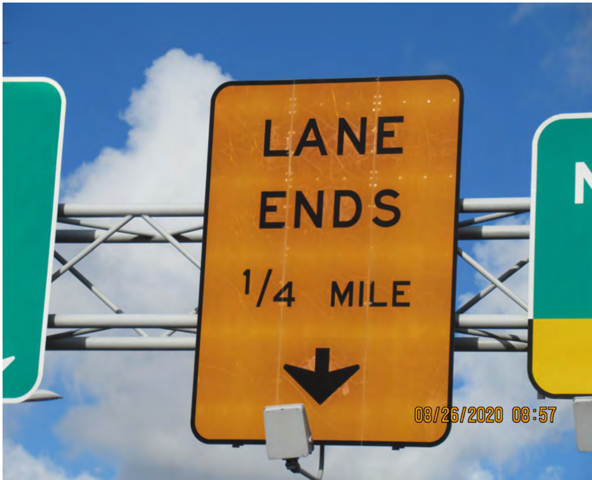
DETERIORATED REFLECTIVE SHEETING ON LANE ENDS 1/4 MILE SIGN PANEL
