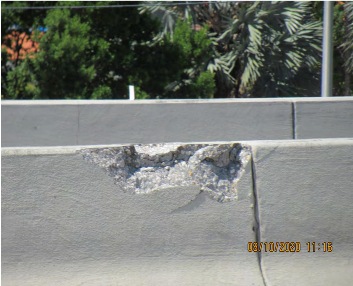
DAMAGED MEDIAN BARRIER WALL (BRIDGE # 870708)
