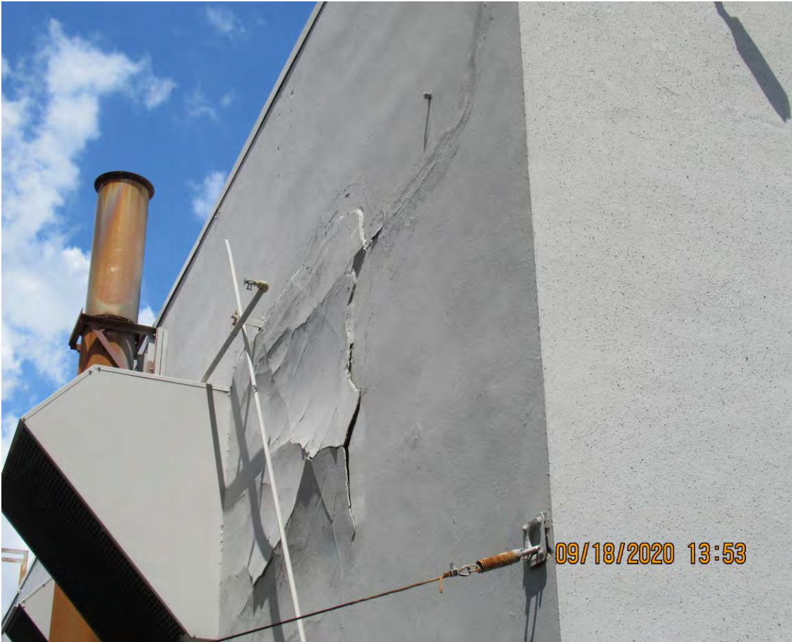
DELAMINATION OF STUCCO (EAST ELEVATION)
