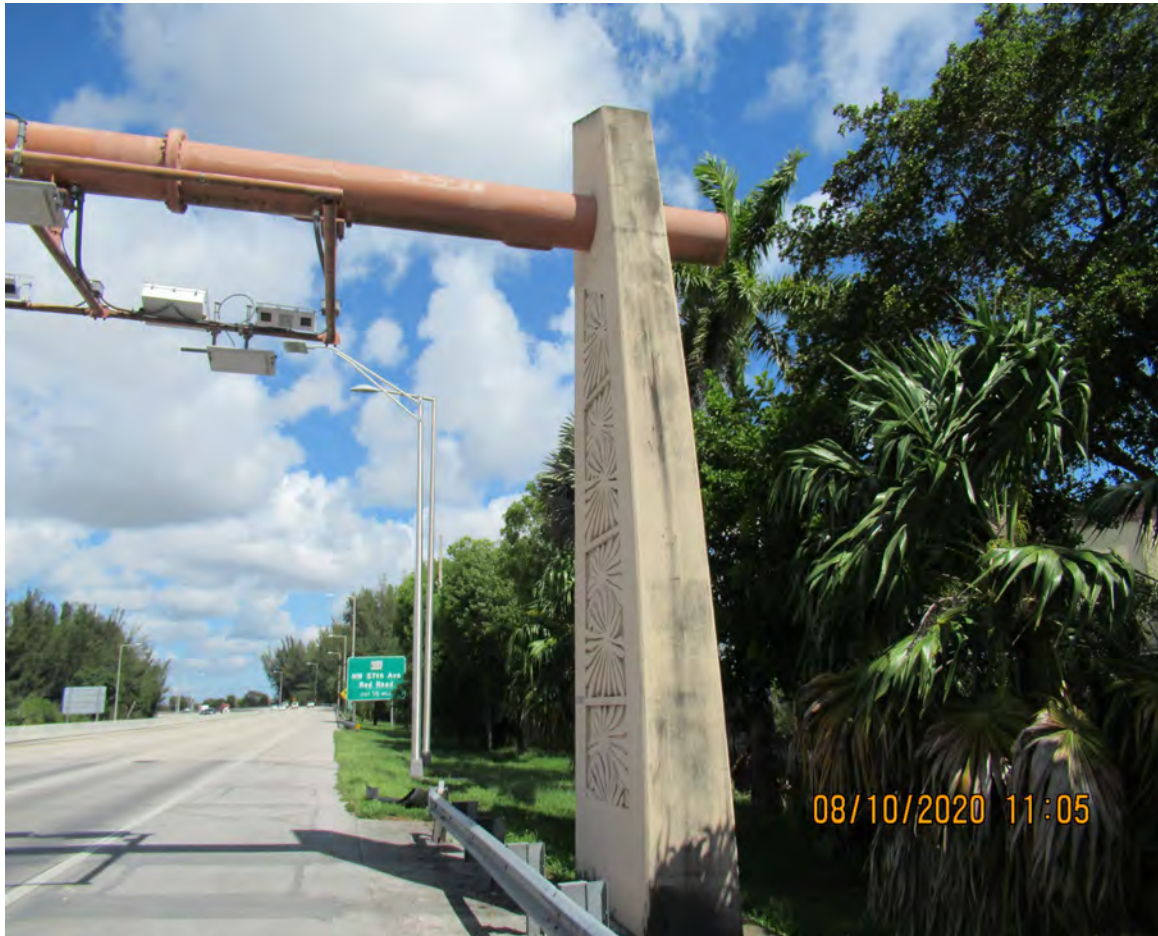
DETERIORATED PAINT ON STRUCTURE UPRIGHT AND MONOTUBE (STRUCTURE # 87S932)
