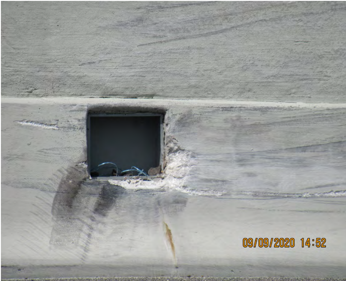
DAMAGED MEDIAN BARRIER WALL AND MISSING COVER ON PULL BOX
