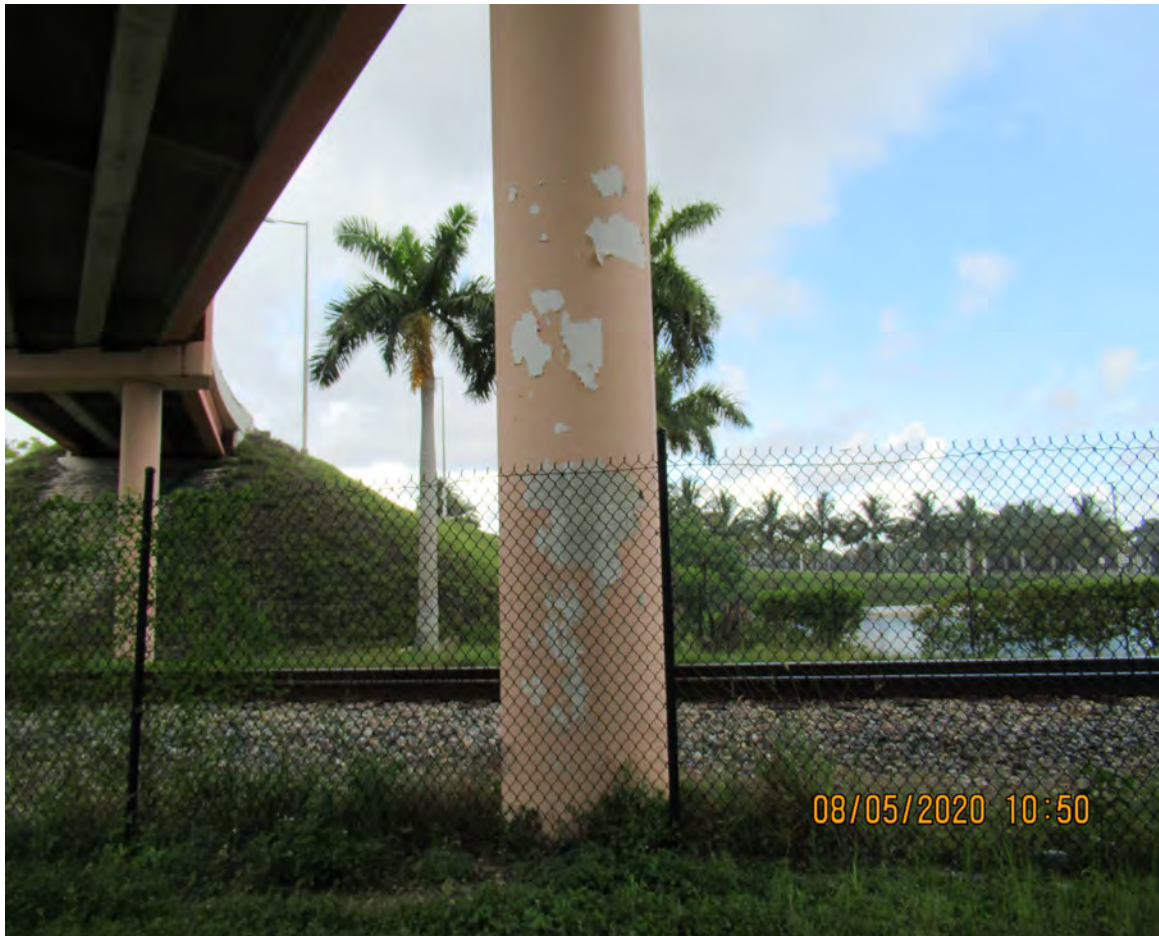
DETERIORATED CLASS V COATING ON BRIDGE STRUCTURE (BRIDGE # 870543) TYPICAL THROUGHOUT THE CORRIDOR
