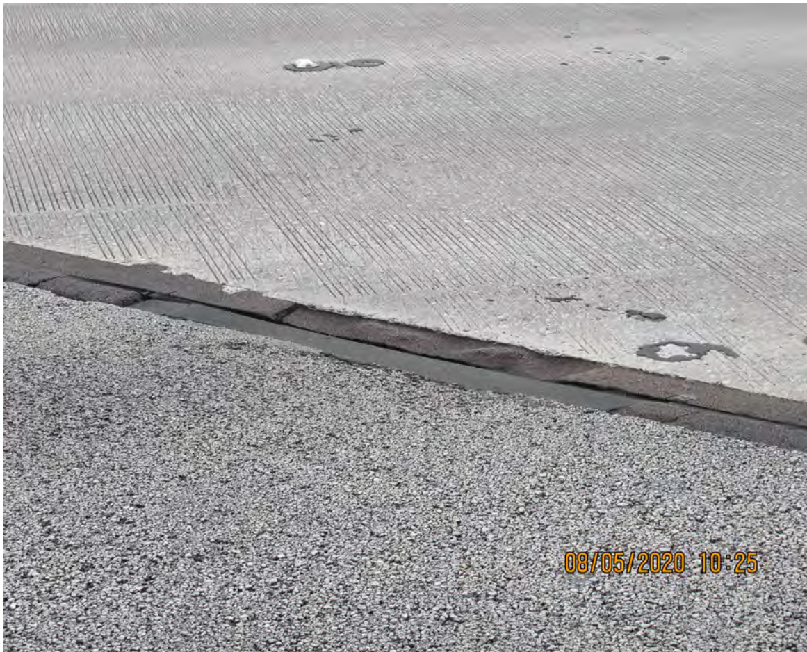
DETERIORATED POLYMER NOSING BRIDGE JOINT HEADER (BRIDGE # 870522)
