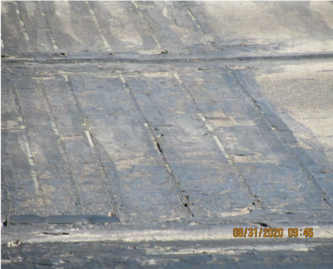
DETERIORATED TOLLS LOOP DETECTOR SEALANT
