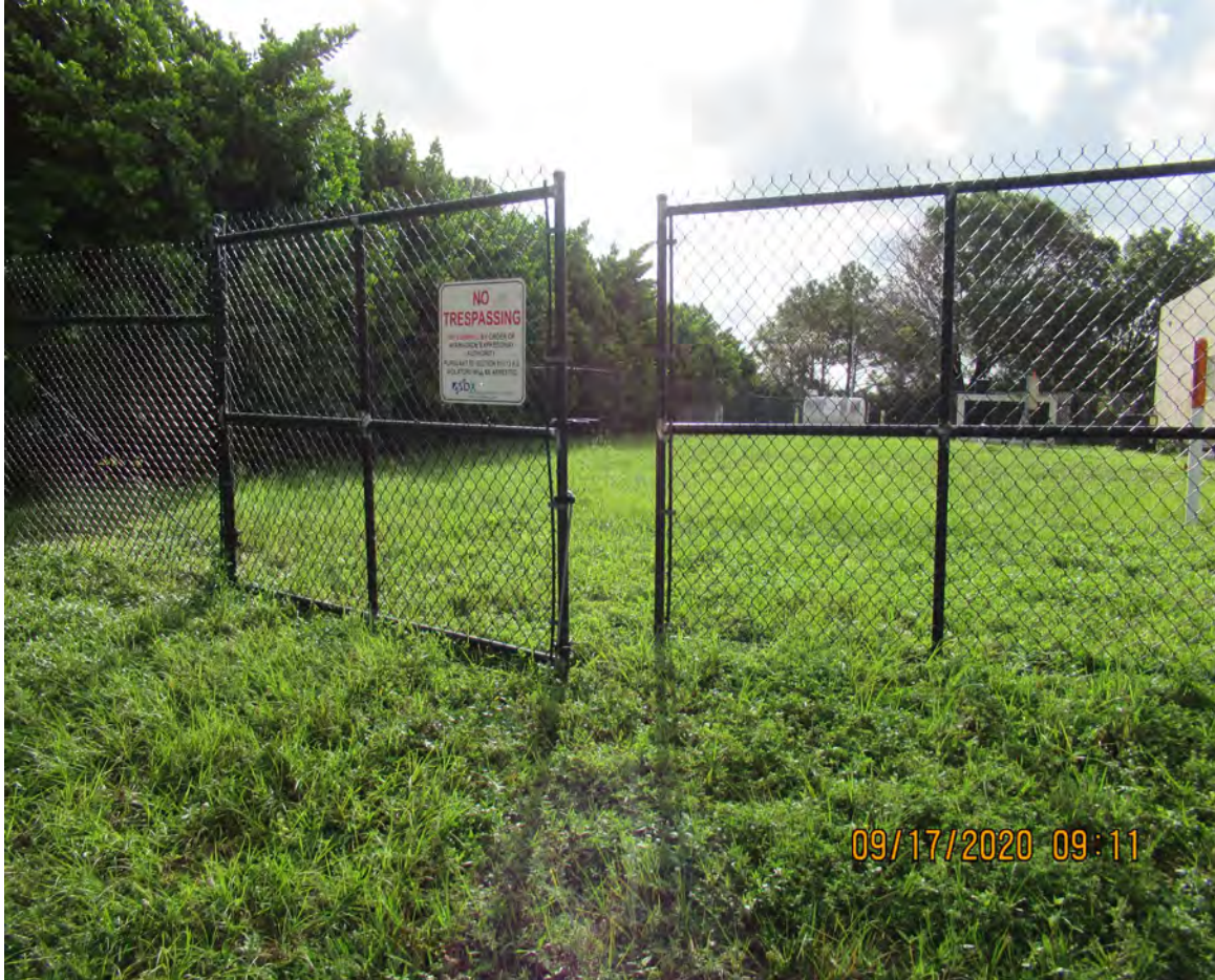
MISSING LOCK ON GATE
