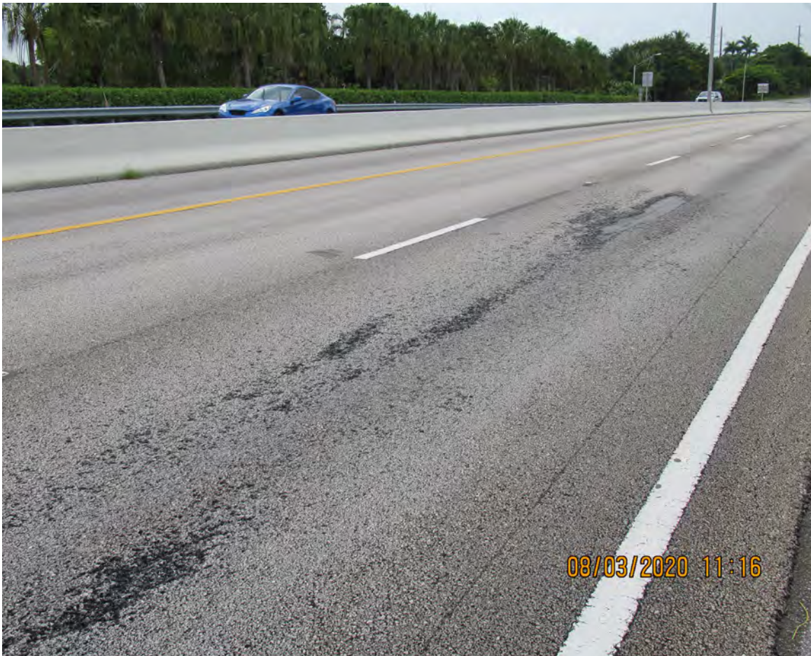
DETERIORATED ASPHALT PAVEMENT
